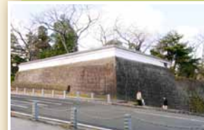
2 Otemon Gate North Earthen Wall (extant)
