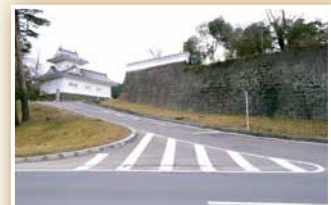
1 Site of Otemon Gate and Waki-yagura Watchtower (reconstruction)
