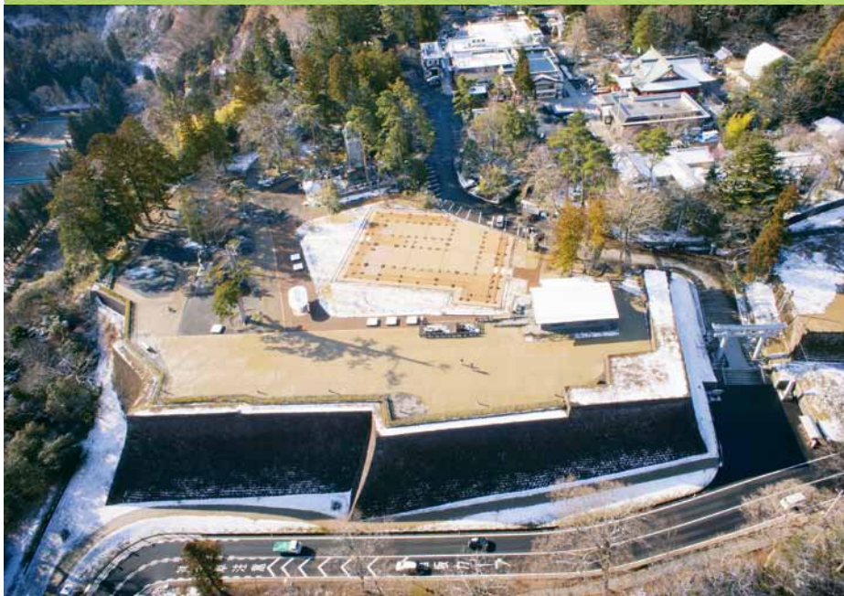
Main Compound's North Stone Wall The Remains of the Ohiroma Large Hall in the Main Compound
