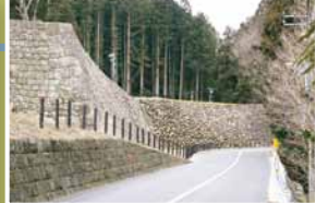
6 Main Compound Northwest Stone Wall
