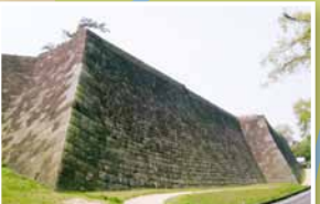
4 Main Compound North Stone Wall
