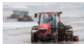
Salt removal work continued in spite of bad weather.
