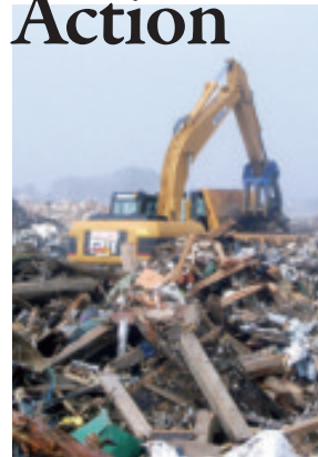
Removal of debris with heavy machinery was extremely difficult.
