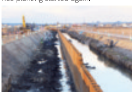
Restoration work advanced steadily.
